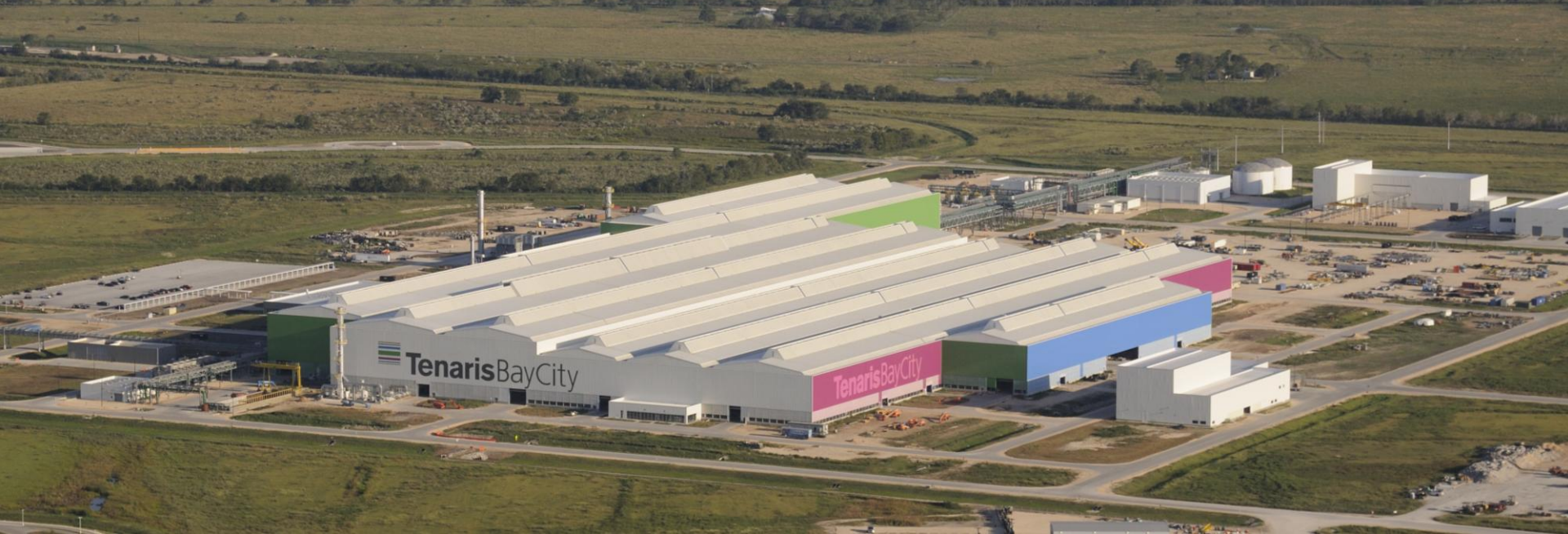
TenarisBayCity Seamless Pipe Mill, US
